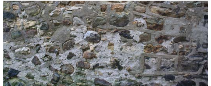
Above: magnesian limestone neatly re-pointed in lime Below: smeared and strap pointing in cement is harmful
