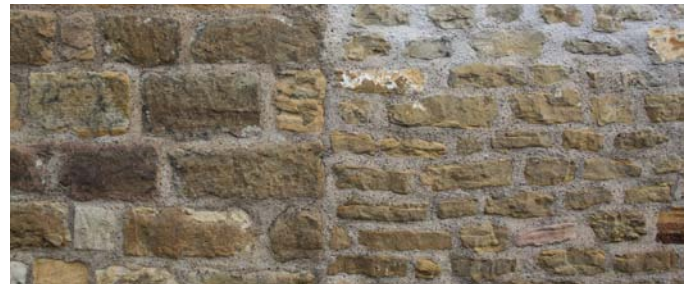
Above: magnesian limestone neatly re-pointed in lime Below: smeared and strap pointing in cement is harmful
