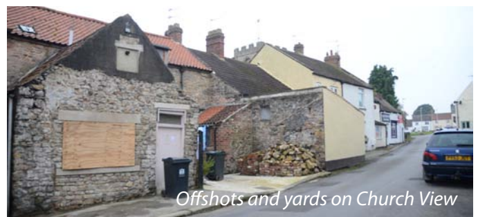
Historic outbuilding north of Church View
