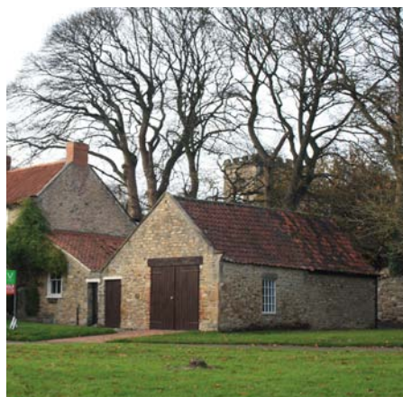
Boundary walls and outbuildings are numerous, adding great historic integrity to the area
